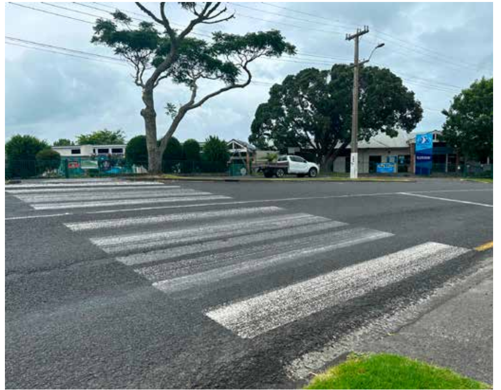
The pedestrian crossing on Maraetai Drive will be upgraded this year.
