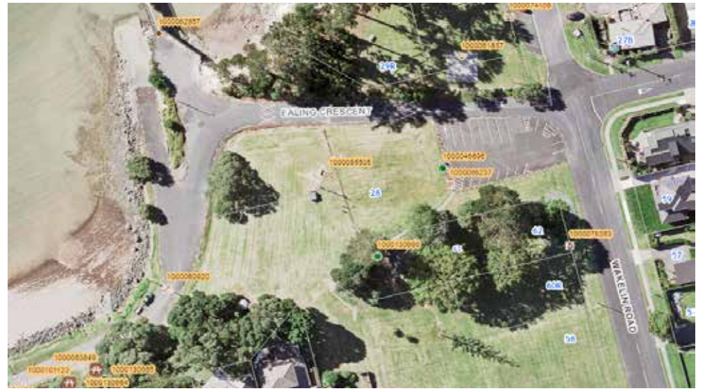
Aerial view of Sunkist Bay, where works will soon be underway to replace degraded infrastructure. Photo / Auckland Council.
