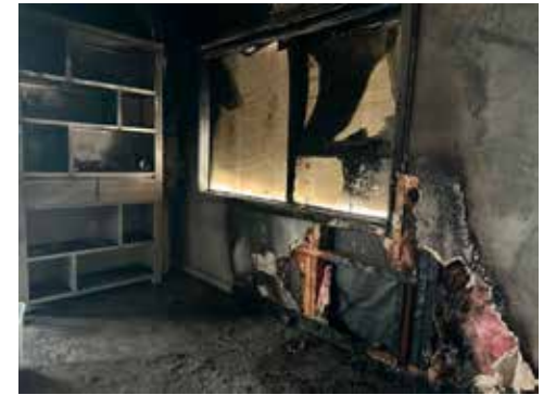
Picture of the living room where a charging lithium battery caught fire.
