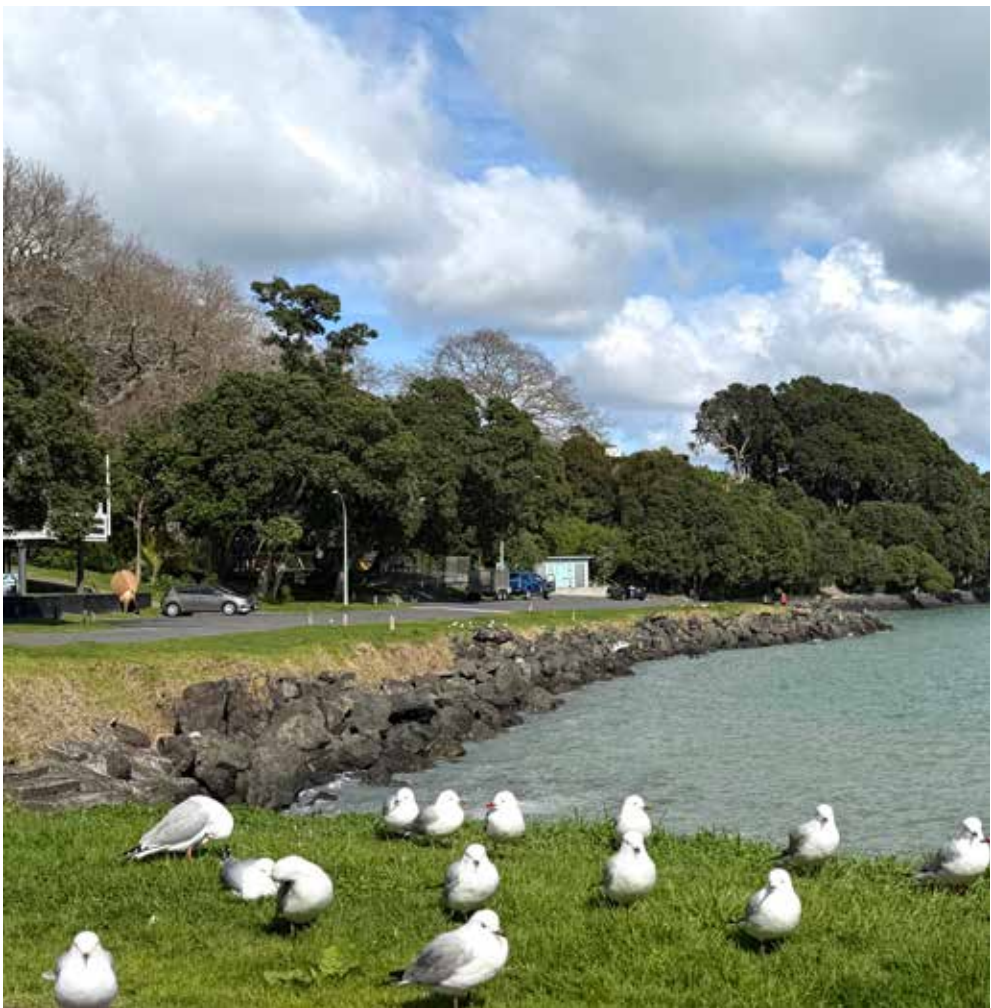
Council is in discussions with a contractor about the Sunkist Bay seawall repair.
